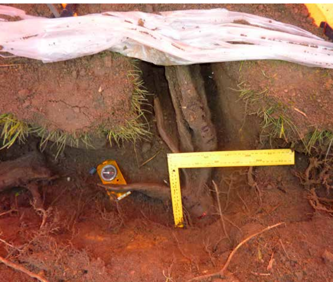
Figure 3 The damaged root section.
